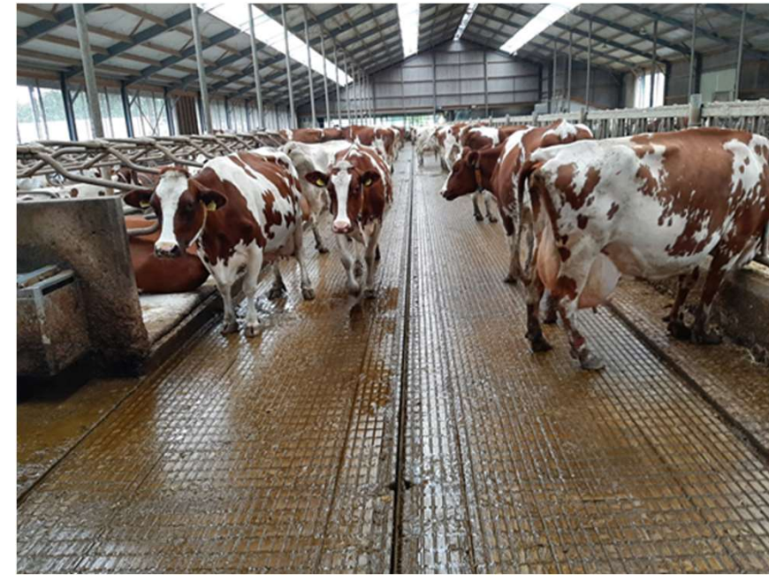
Concrete separation Floor, farm van Boxtel
