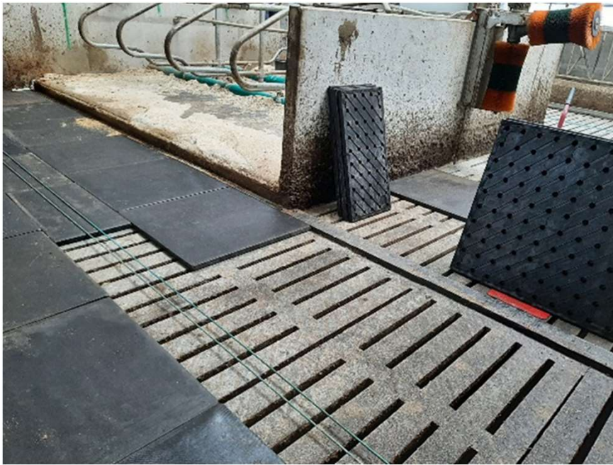
Permeable floor (ZeraFlex), Dairy Campus
